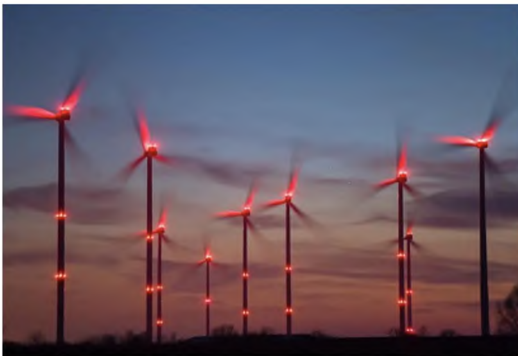
Figure A3.3-2 Red obstruction lights in the "Odervorland" wind farm in Germany
